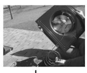
I: Apply sealant to bottom edge of panel flange, tucking upper flange under shingles. J: Fasten panel to roof using 4-8 screws. K: Bring wire to fan opening.
