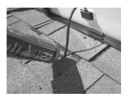
E: Find south or west-facing roof to mount panel, and drill 3/8'-1/2" hole through roof. F: Connect ext cord to panel cord. G: Feed wire into attic. H: Seal hole.
