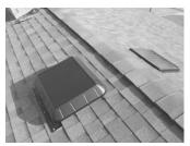
M: Slide fan under shingles. N: Center fan over hole. O: Screw fan base to roof. **P**: Installation complete - The Sun's **FREE** power is now cooling your attic!
