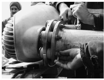
Fig. 10 Grounding turbine to tower
