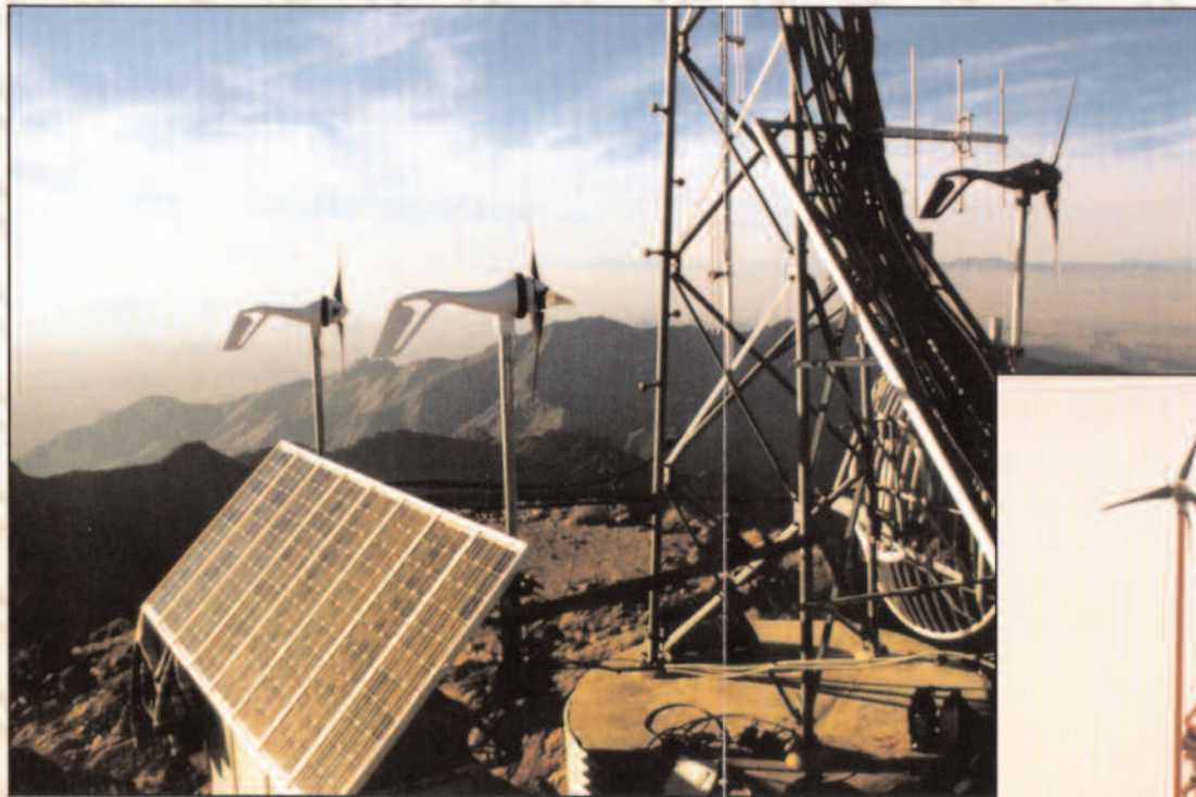
Three Air Industrial modules combined with PV provide power for a cell phone transmitter in the mountains near Phoenix, Arizona.
