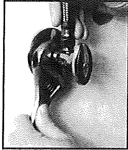
1. Turn off water supply and remove angle stops.
