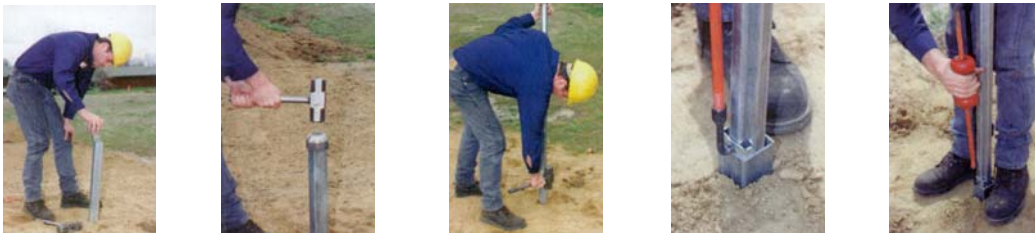
Figure 3: Nex® Sign Support System Installation
