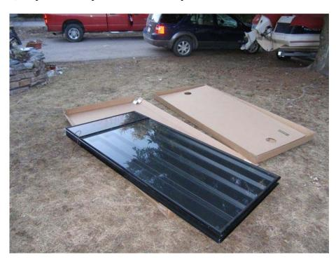
2) Find the location where the SolarSheat will be mounted. The location should be due south. You can use a compass or watch the sun strike your building during sunny
