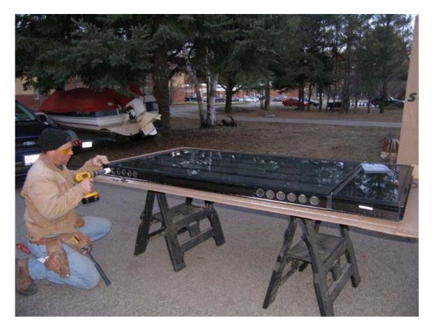
9) Cut and position the pieces of EPDM foam included with the duct kit above and below both sets of holes. This is for sealing the channel for airflow and will prevent the air from leaking into the rest of the SolarSheat channel. Refer to owners manual for foam placement.
