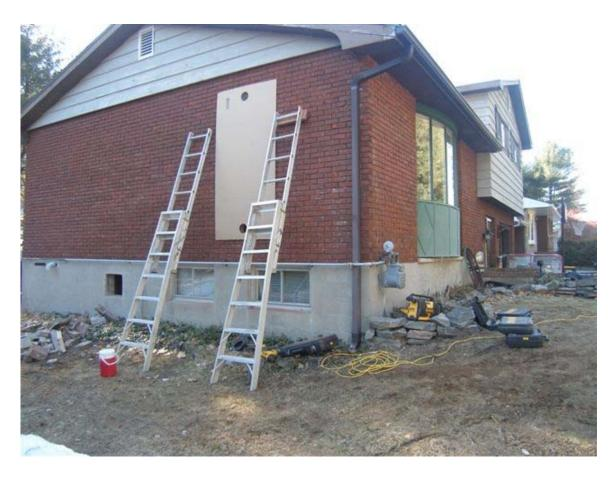
4) Next use a core drill 5" or large drill bit to breakthrough the brick or siding.
