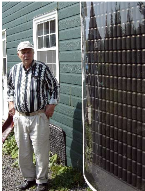
Above: Consolair's SolarMax collectors incorporate 240 aluminum cans.
