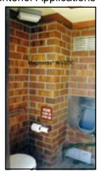
This unit is controlled by a motion sensor set for 30 seconds. Listed UL® "Wet Location", and bug/dirt proof.
