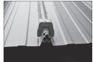
Example of correctly installed S-5-KHD clamp
