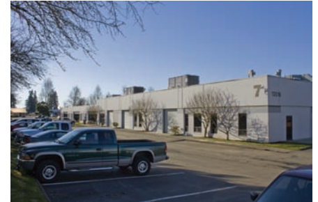
Silicon reprocessing - Vancouver, WA
