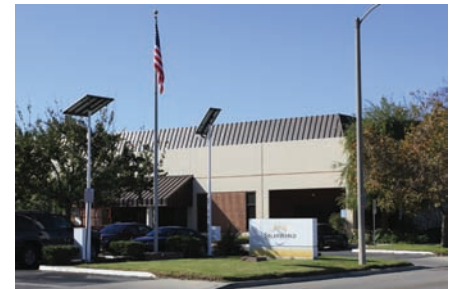
Module assembly and sales center for the Americas - Camarillo, CA
