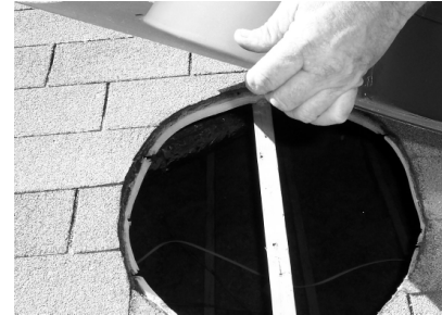
Figure 2 - Cutting the Vent Hole
