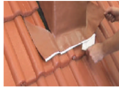
Figure 1 - Bottom Flashing
