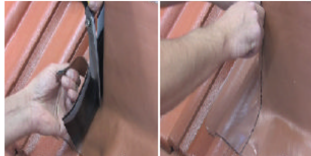
Figure 2 - Side Flashing
