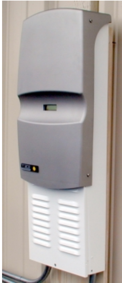
Figure 10 Replace Outer Cover and Screws
