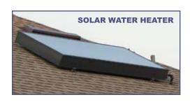
SOLAR WATER HEATERS provide instant hot water from a collector on your roof that is heated by the sun and a storage tank (your current or an additional water heater). This hot water can be used for showers, washing machines, dishwashers and in the kitchen sink. The SWH purchased by the Santiago Family provides up to 90% of the family's hot water needs.
