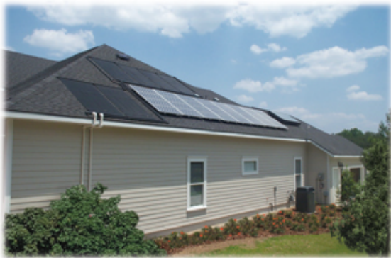
Image above shows from left to right: solar pool heater, solar electric system and solar water heater. Systems can be installed on roof or ground rack.
